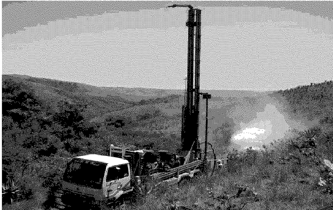
RC Rig on site 8 th December 06
